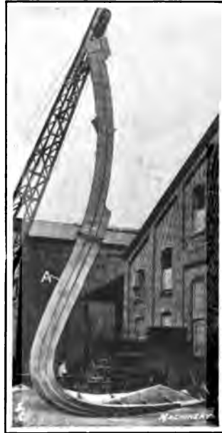
Fig. 3. Steel Casting for the Bow of a Ship
